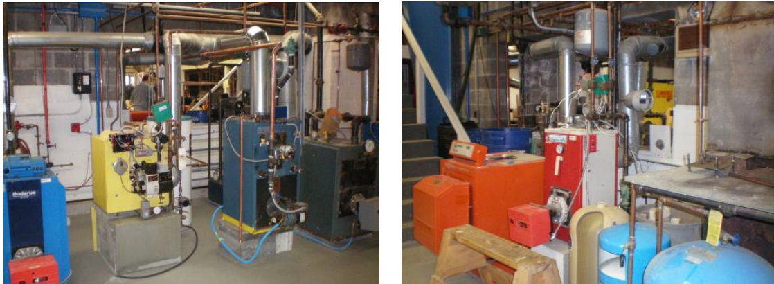
Mock Boilers and Furnaces Flue Gas Exhaust Pipe
