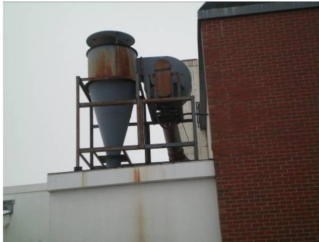
Residential Construction Dust Collector
