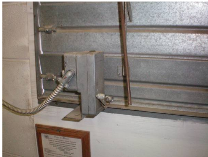
Commons' Combustion Air without Linkage
