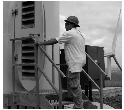
Ryan Fonbuena, operations manager for First Wind, the company that runs the Mars Hill Wind Farm, stands at the base of one of the turbines on the Aroostook County mountain. Currently the largest wind power production facility in Maine, the Mars Hill project will benefit from the wind power technology program that will begin next year at NMCC.
