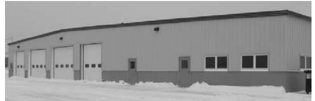
Future site of the Northern Maine Center for Excellence in Alternative Energy Training and Education.
