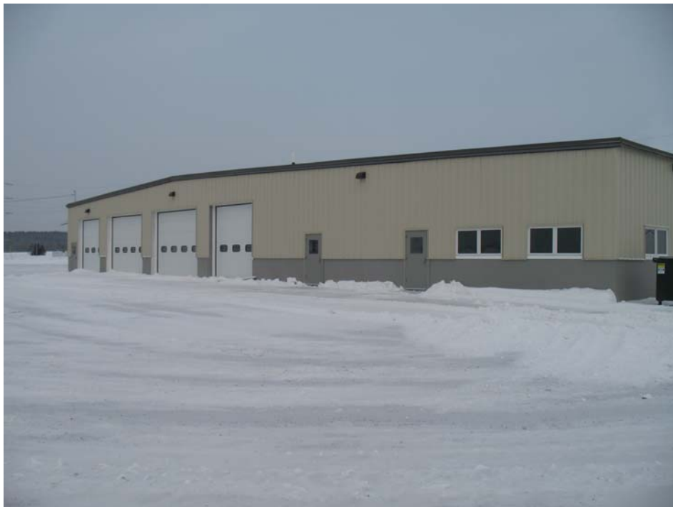
Future site of the Northern Maine Center for Excellence in Alternative Energy Training and Education.
