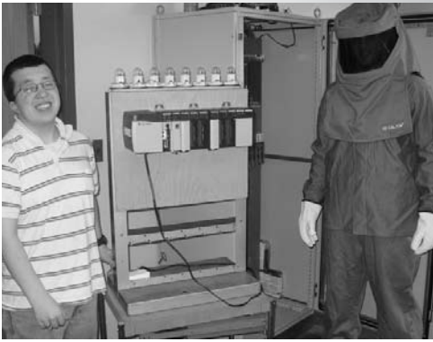
Students Jared Reed of Washburn (left) and Lance Getchell of Milford (in arc flash gear) are two of the many students in electrical and electronics related programs at NMCC that are benefitting from the donation of equipment by Twin Rivers Paper Company of Madawaska. Featured in the photo between the two students is the programmable logic controller donated by Twin Rivers and the arc flash gear suit (worn by Getchell) also donated by the company.
